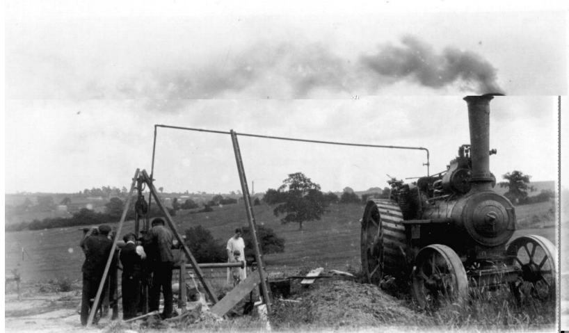
Drilling a 70ft well at Blisworth Cannock 1924 at house of John and Winifred Millar
